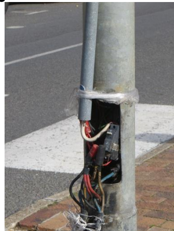
Figure 39 Street light poles with no electrical covers
